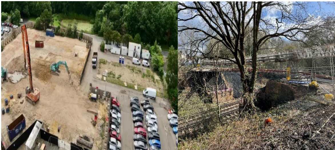
Demolition of the old hospital buildings
